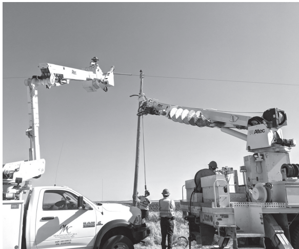
Lineworkers perform a hotline changeout and pole top rescue
